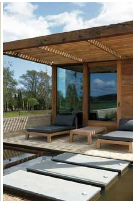
Operable windows in solid French oak finished in water-based lazure, leaving the pores of the wood open.
